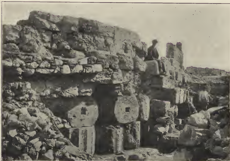
FIG. 12.—Architectural Fragments of the Old Athena Temple built into the North Wall of the Acropolis.
